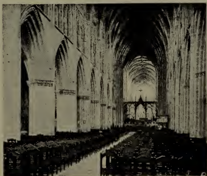
NAVE, LOOKING EAST.
